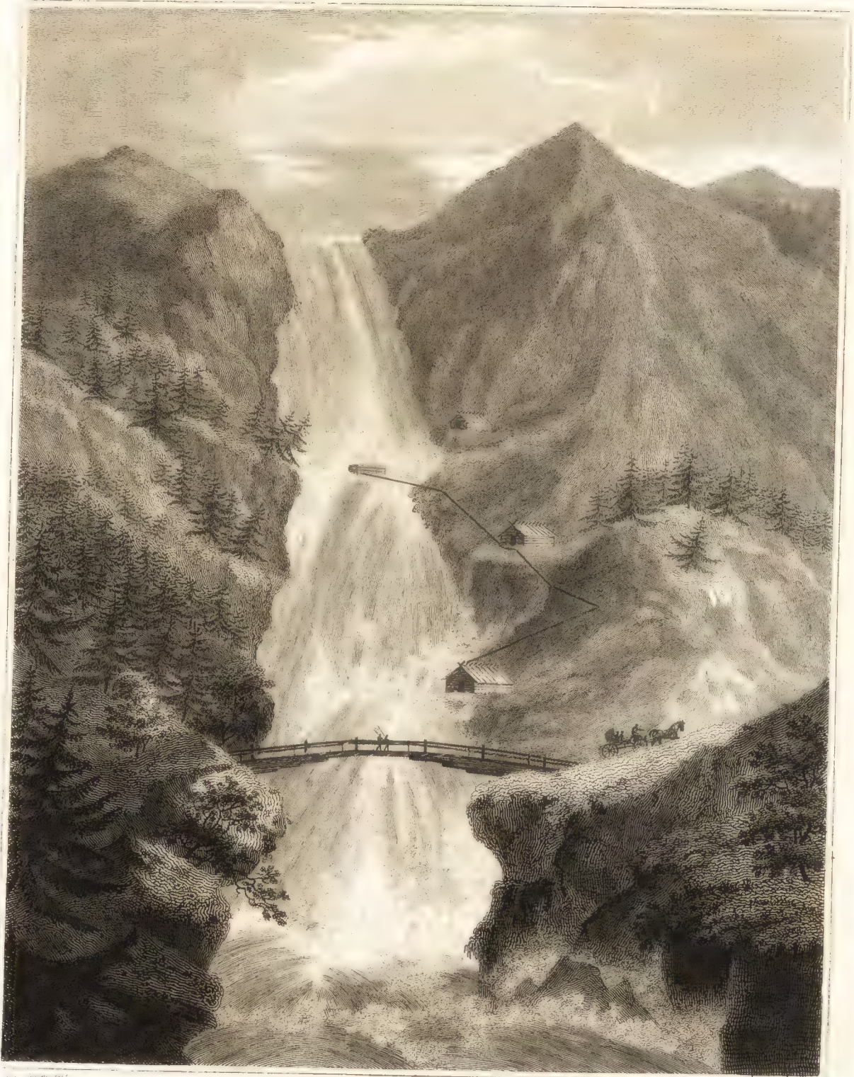
CASCADE, and BRIDGE constructed of the Trunk of PENNA.
